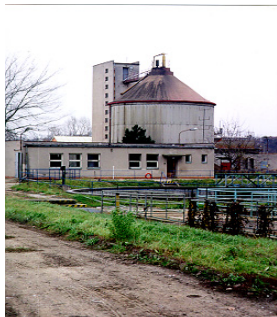
Fig 2 Wastewater treatment plant in Břeclav
