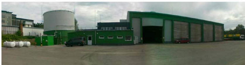
Figure 3 Biogas plant in Žďár nad Sázavou
